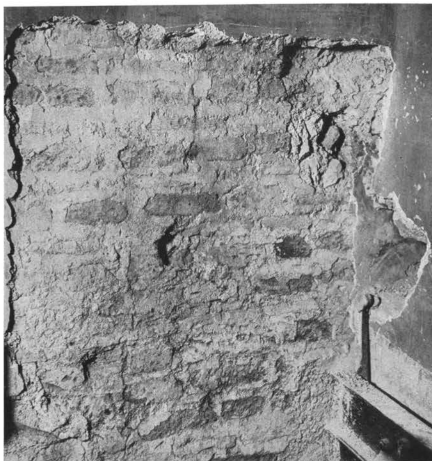
Fig. 145 — S. Lorenzo in Lucina. Opus listatum in the east wall of chancel (Photo: Sansaini).
